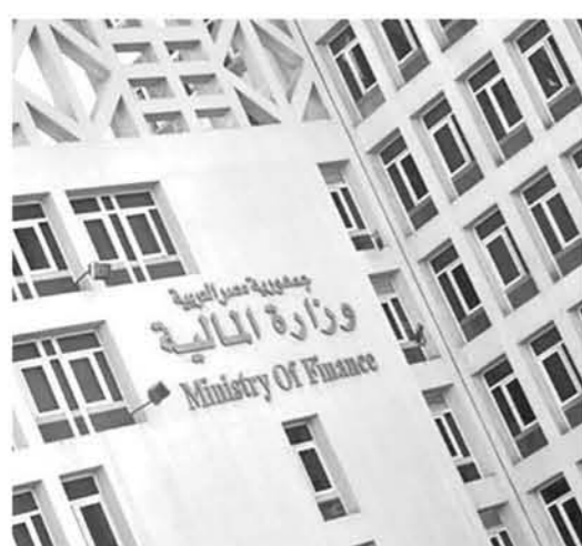
Headquarters of Egypt's Finance Ministry
